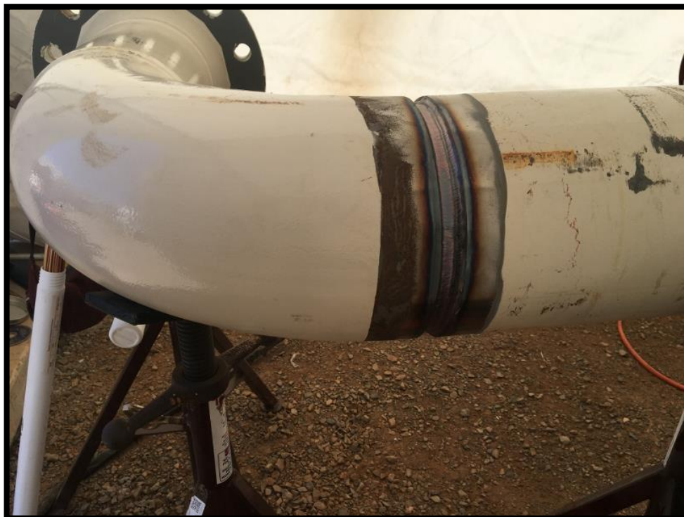
Inlet Station – Welding of 8" Kicker line FWW
