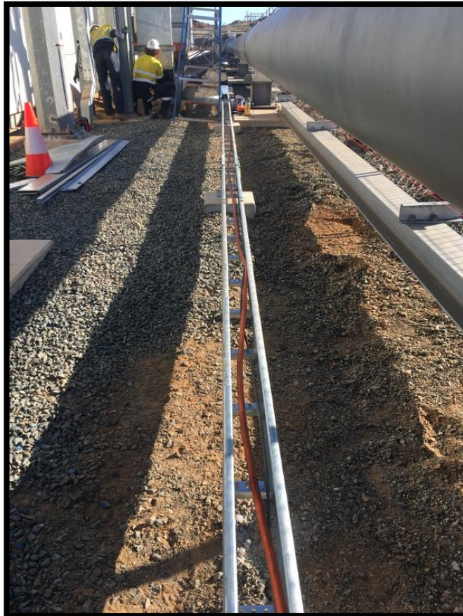
Inlet Station – Tray & cable installation
