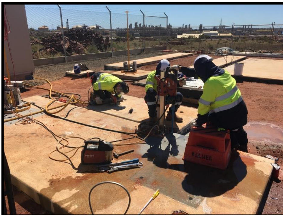
Meter Station – Core drilling and scabbling
