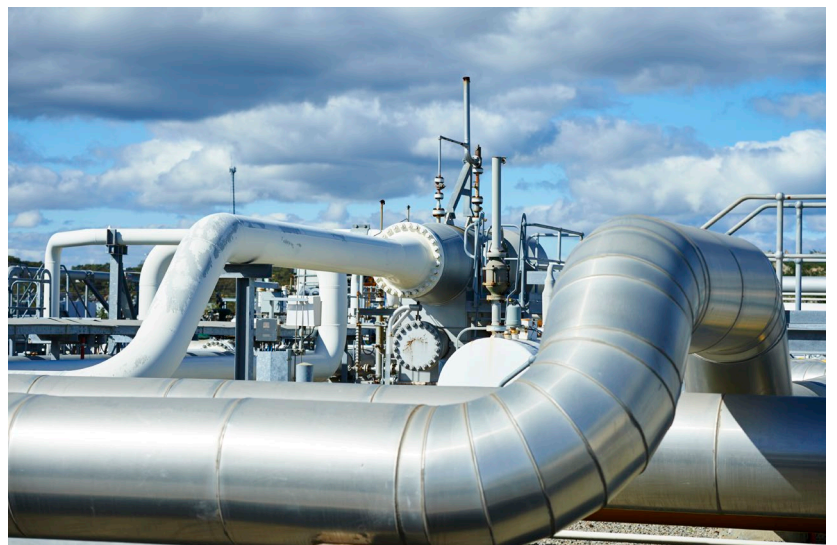
Figure 9.11: Compressor Station 10 in Kwinana
