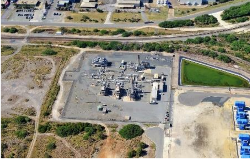
Figure 8.4: Aerial view of Compressor Station 10
