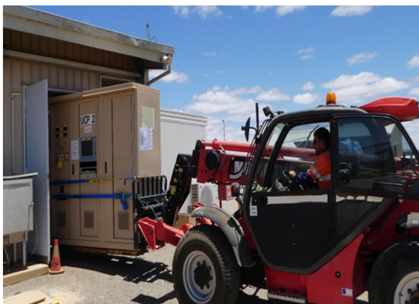
Figure 8.5: Replacement on compressor unit control panel (UCP)
