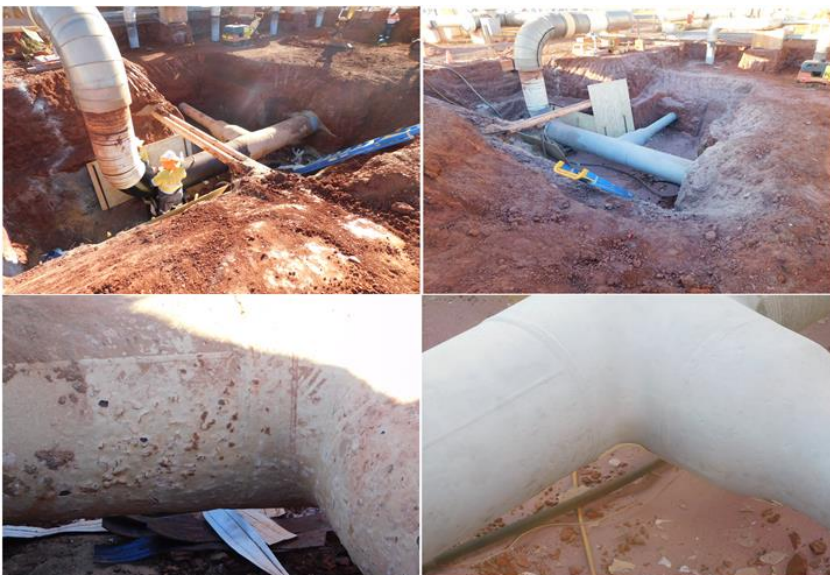
Figure 8.11: Refurbishment of underground piping at CS1
