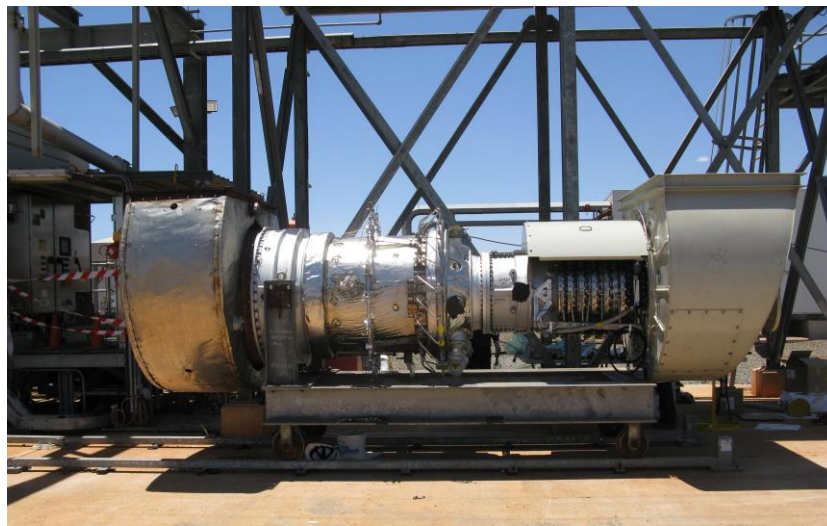
Figure 7.7.4: Turbine exchange, Compressor Station 2, Unit 3, September 2018
