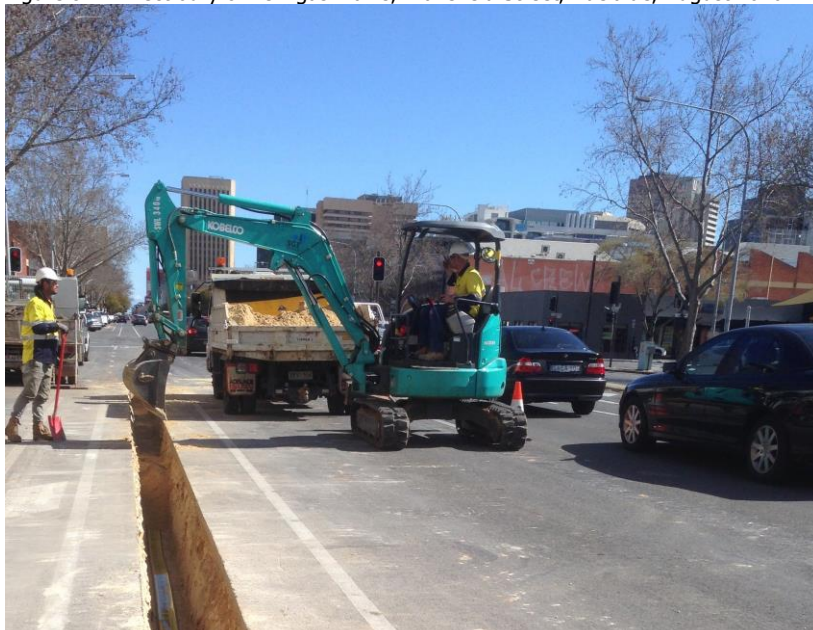
Figure 8.7: Direct bury of new gas mains, Wakefield Street, Adelaide, August 2016
