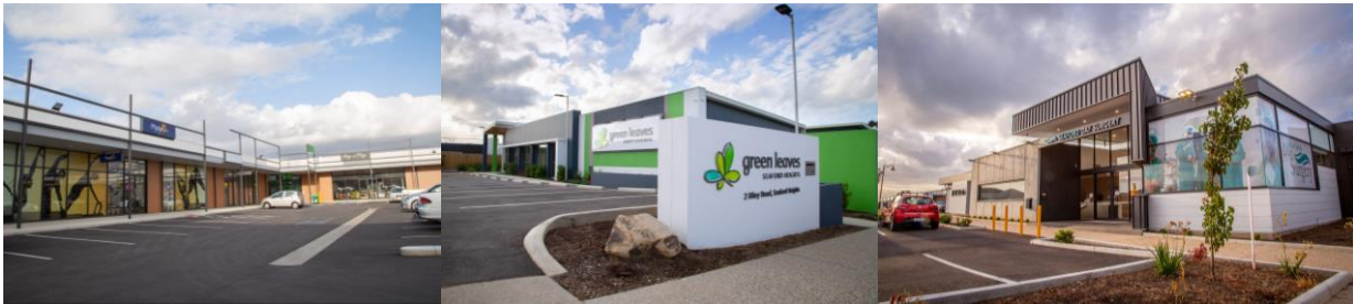
Figure 8.8: New Industrial and Commercial connections at the Vista development in Seaford. Photos courtesy of the UDIA SA.
