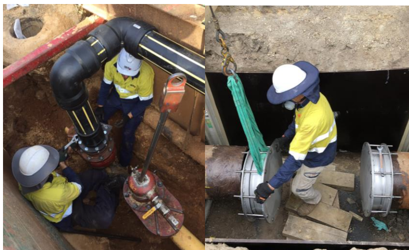
Figure 8.10: (from left) Isolation and bypass on a live steel gas main, South Road, Hindmarsh, April 2017; Cut and capping low pressure cast iron main, Grote Street, Adelaide CBD, October 2016
