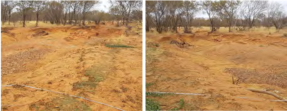
Plate 1: Erosion recorded at site 6 – rehabilitation plot
