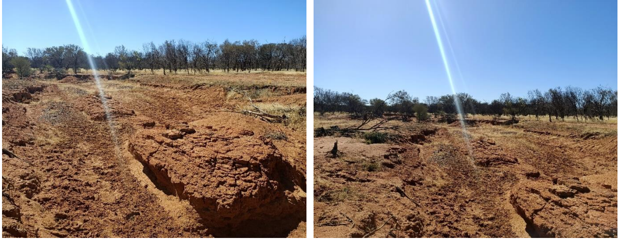
Plate 1: Erosion recorded at site 6 – rehabilitation quadrat
